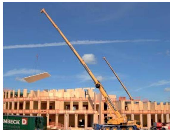
Figure 7: CLT panels being lifted into position – construction should be fast compared with most traditional methods, although additional resources may be needed in the planning and design stages
