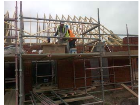
Scheme Apprentices on local housing site
