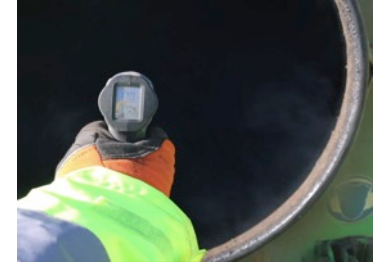
Heated & mixed for 6-10 minutes until the the mix reaches 170°C
