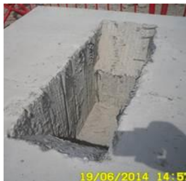
Image 2, bolt pocket after pouring concrete and removing temporary form.
