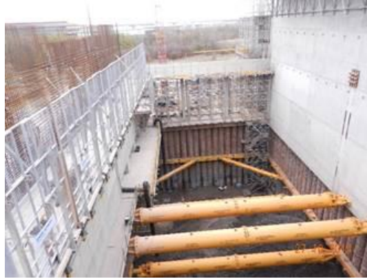
Image 5, showing walls above ground progressing prior to lower wall commencement
