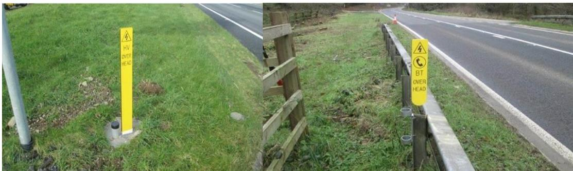
Attention was then turned to the way it would work by a VRS fence (Vehicle Restraint System) and it was decided to mount the blade to the post of the safety fence similar to the marker posts already in use on the Trunk Road network.
