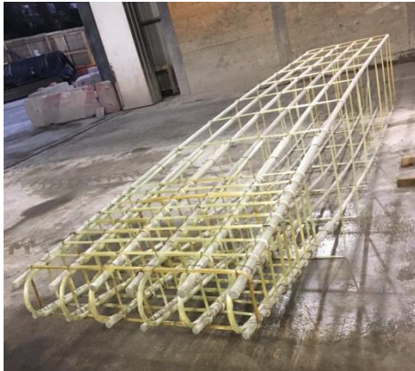
Figure: Preassembled GFRP cage
