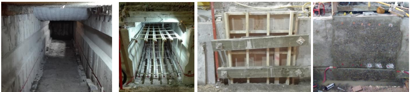
Figure: Invert concrete works from excavation to installation to concreting.
