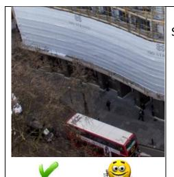
Sheeting/netting will comply with BS 7955 1999 and be fitted to BS 8410 2007 to the outer facade of the scaffold At no time may sheeting be left loose and unsecured
