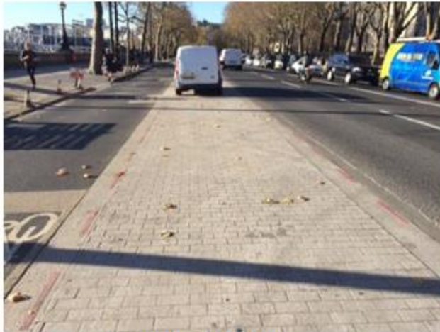
Victoria Embankment works location
