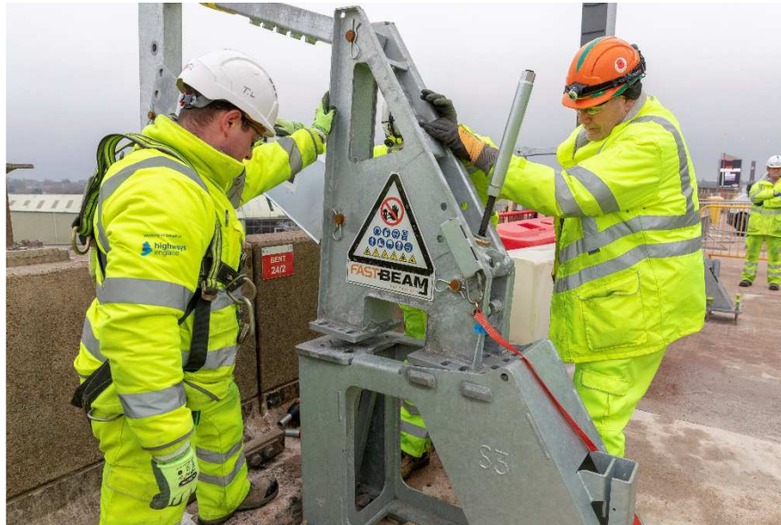
Craning the working platform into place.
