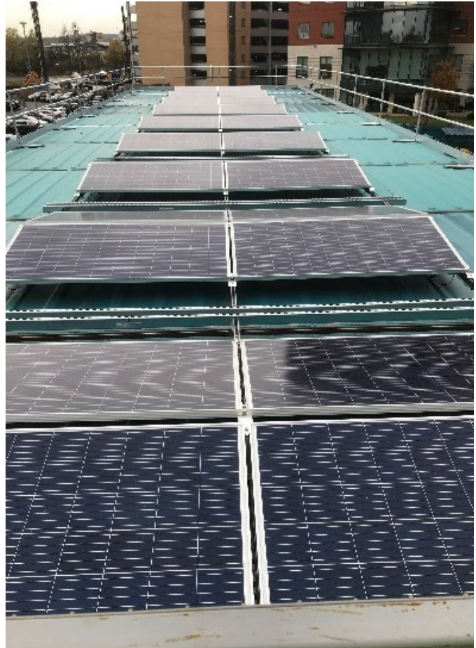
Figure 15: Solar Panel Array
