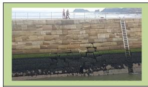
East Pier: section of wall requiring repair to face
