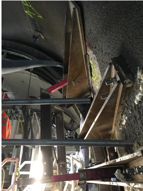
Photo 1.6 Handling frame in operation while placing the bracket into position
