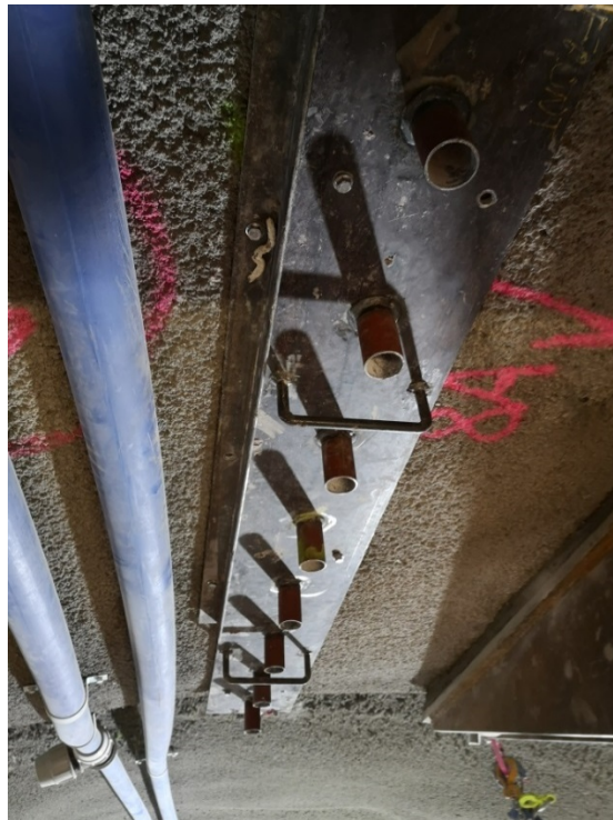
Photo 1.5 Holes Drilling Template
