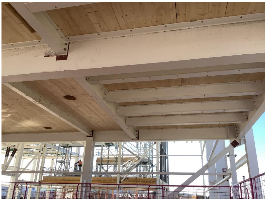
CLT slab from below
