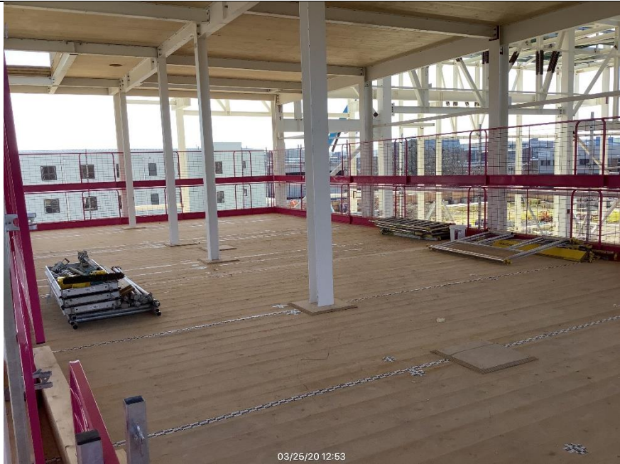
CLT slab from above
