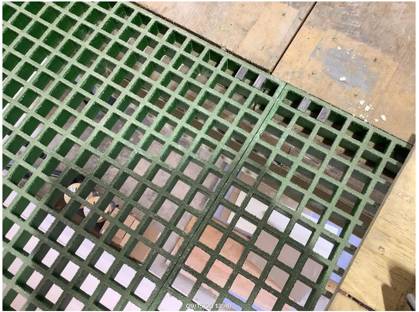
CLT GRP riser interface
