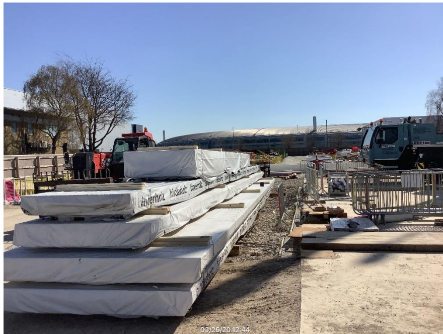
CLT shipped to site wrapped to ensure clean and dry
