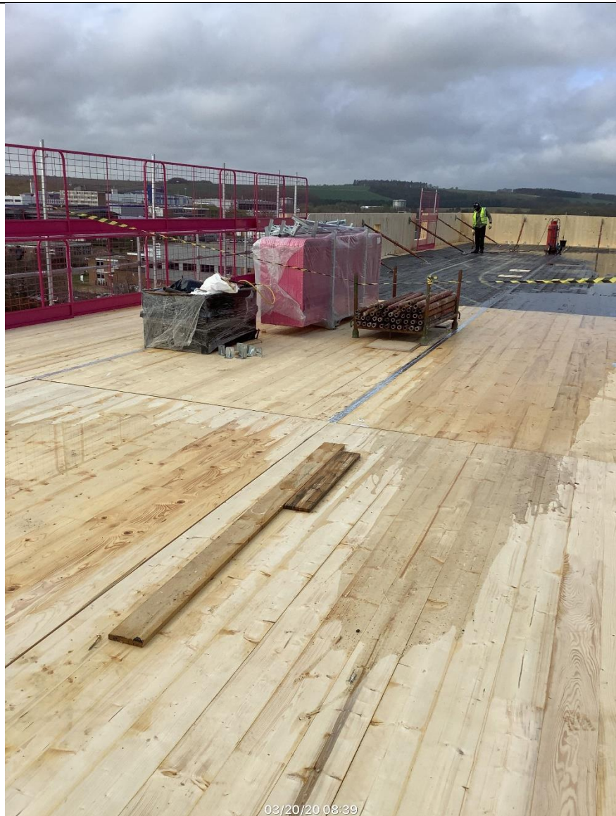
Roof finishes installed directly onto CLT
