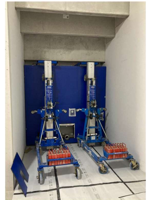
2No. Genie's During Site Installation with limited headroom.
